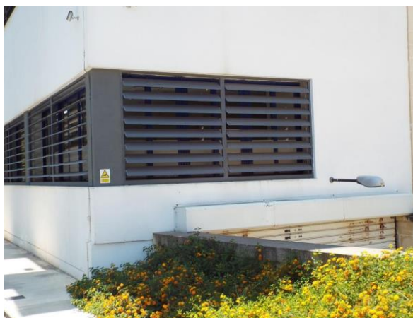
Figure 2 External shading helps the spaces remain cooler by keeping sun's rays from entering inside.
